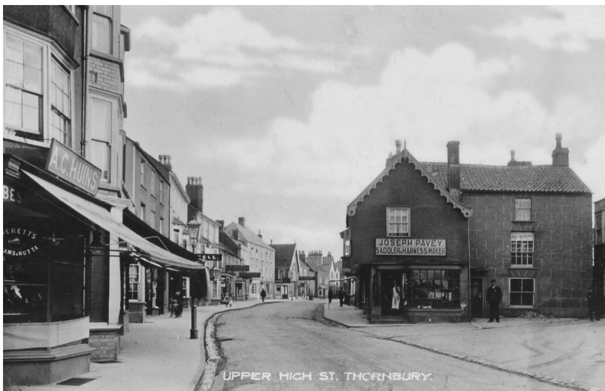
Historic pinch point early 1900s
